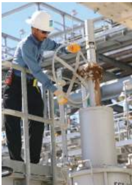
Rig incidents have directly led to tightening up of regulations and improving working practices throughout the industry.
