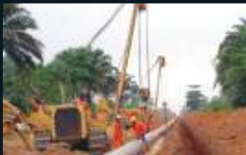
The Umugini pipeline under construction.
