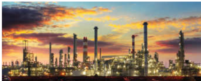
AllAssets 3.0 is the latest major update to the solution, due to roll out to customers in March 2022. The cloud-based software has been customers reduce risk of asset failure by up to 95%.
