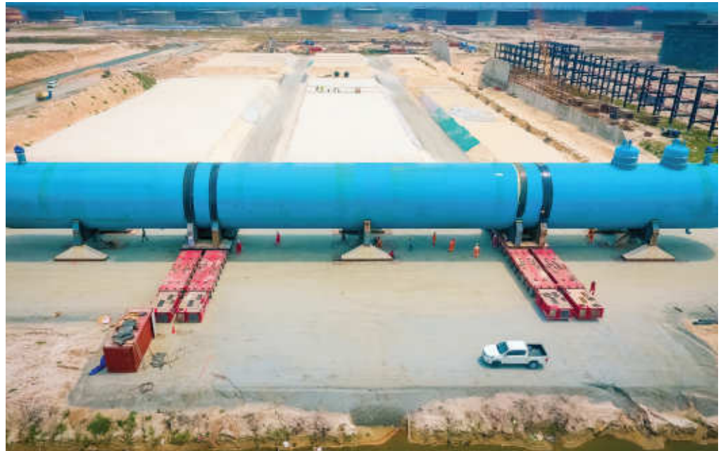
Installation of LPG bullet.
