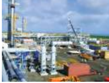
The US$180mn gas engine-driven power project takes off in Ghana.
