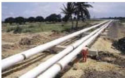
Pipeline carrying natural gas from Mozambique to South Africa.
