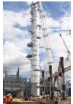
Construction has begun on the world-class furnaces and aboveground piping systems.
