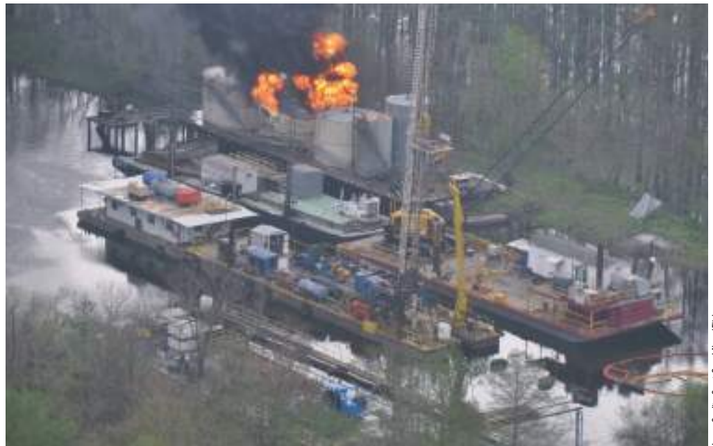
A platform caught fire in Bayou Sorrel, Louisiana, in March this year while in the process of being dismantled.
