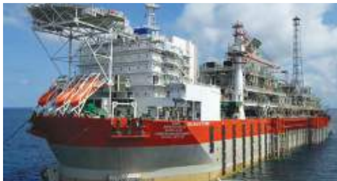
BP's Greater Plutonia FPSO - Phase III is slated for near-term completion.
