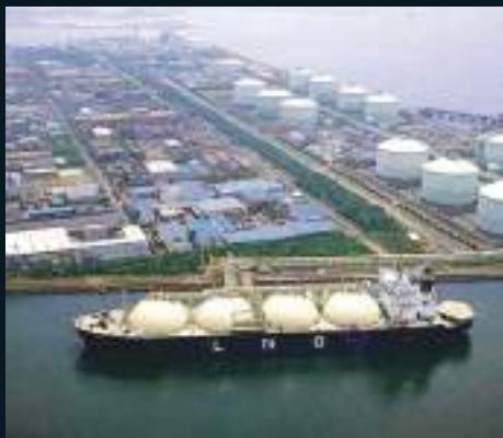
BW Gas is to provide Egypt with a floating LNG terminal.
