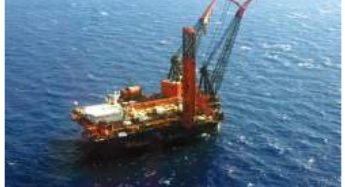
Remaining on the FID list is the Total-operated Kaombo Project.
