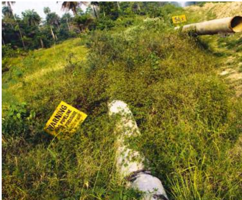
Poor pipeline maintenance is an example of poor economic management when cost-effective repairs can be made.
