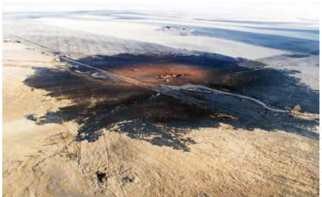
Failure to detect leaks can ultimately result in rupture or explosion. This is the Cabri pipeline in Saskatchewan, Canada.
