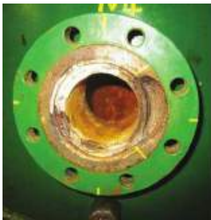
4" flange before and after composite repair.
