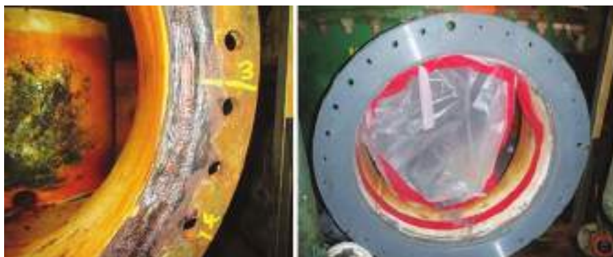
24" flange face before and after composite repair.
