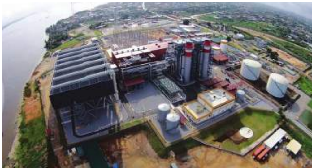
An aerial view of the recently completed Azito complex thermal power plant in the Côte d'Ivoire by Hyundai E&C.
