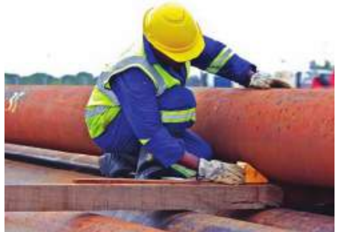
Anadarko has selected a consortium consisting of CB&I, Chiyoda and Saipem (CCS JV) for the initial development of the onshore LNG park in Mozambique.
