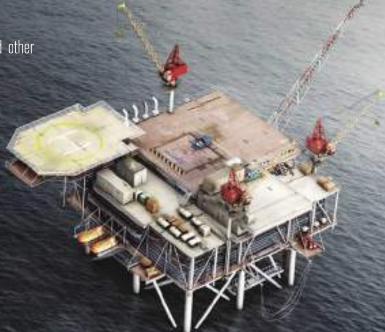
AccessESP installed the first rig-less ESP conveyance system in Nigeria.
