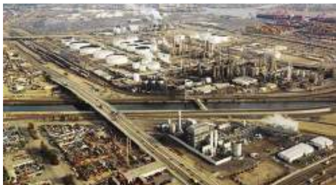
There are many different types of corrosion African refineries are vulnerable to - the Sapref refinery in Durban.
